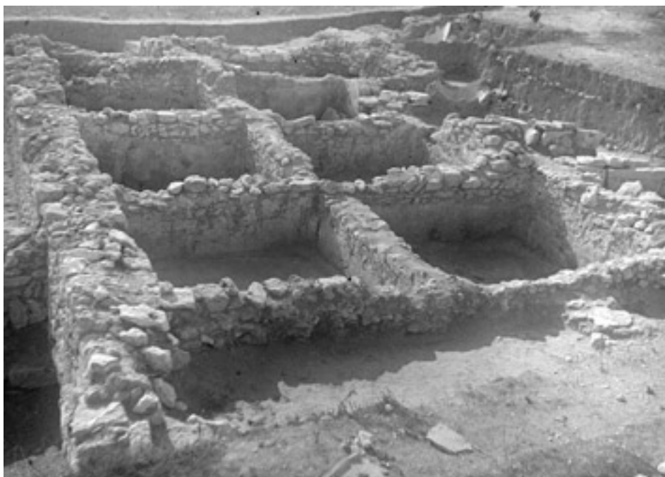
Fig. 11. Salting unit in Myrmekion with a capacity of 116 m 3 (courtesy of the Photo Archives of IIMK RAN).
